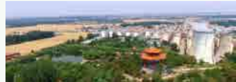
An aerial view of the Xinglongzhuang Coal Mine
