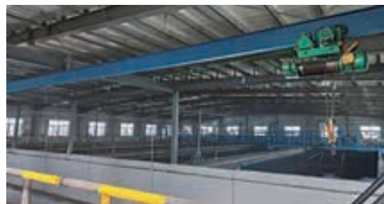
Jinjitan Coal Mine: Mine Water Expansion Project
