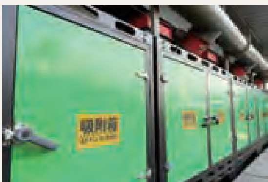
Upgrade of VOCs treatment facilities at the Dongtan Coal Mine
